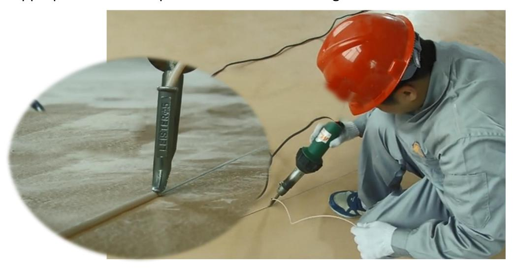
When the electrode is semi-cooled, use the trimmer or crescent spatula to roughly remove the part of the electrode higher than the floor surface; When the electrode has cooled completely, remove the remaining raised parts.
