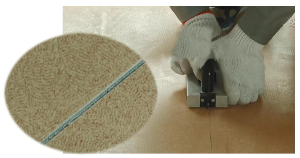
Before welding, the residual dust and debris in the aperture' slot should be removed.
