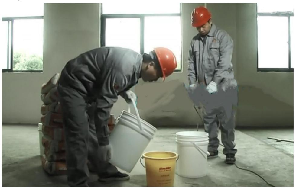
In order to ensure the evenness of self-leveling. It is necessary to use a high-power professional mixer with a mixing head to stir the slurry for no less than 2 minutes until there is no agglomeration in the slurry. Standing for about 1 minute, stirring again.
