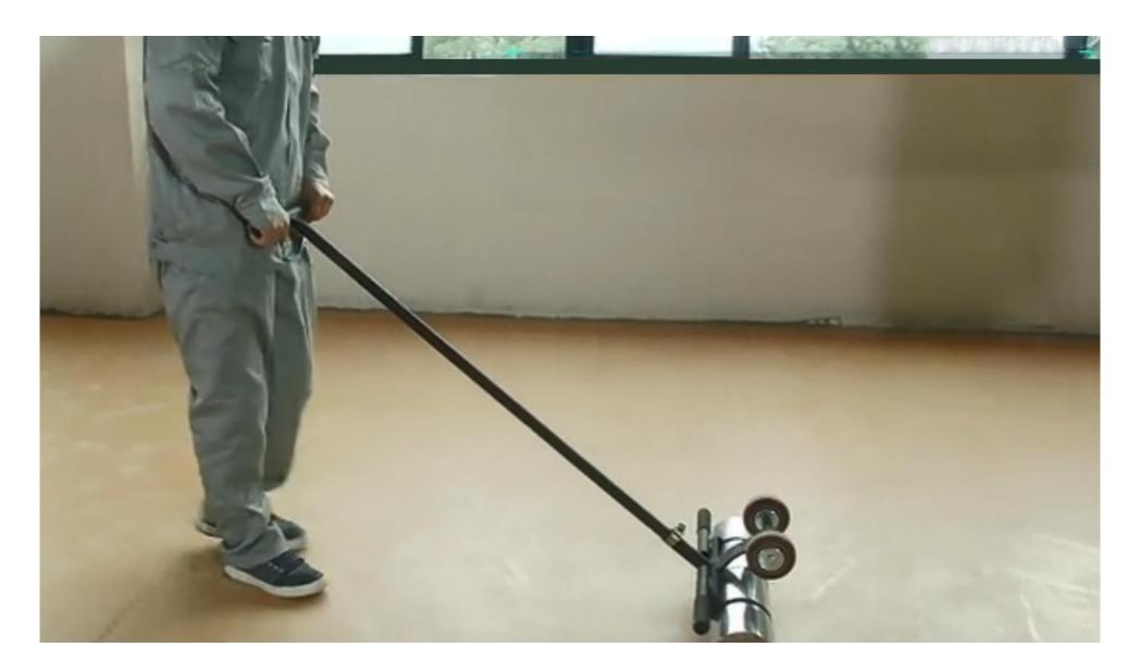
The floor can't be grooved until the glue has fully solidified. Using a special grooving machine to groove along the seam. In order to make the welding firm, the seam should not be permeable. The groove depth is 2/3 of the floor thickness is recommended.
