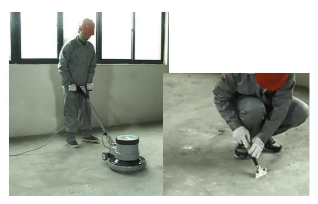
The sanding machine to polish the subfloor with the appropriate grinding disc that is to deal with uneven surface and floating ash.
