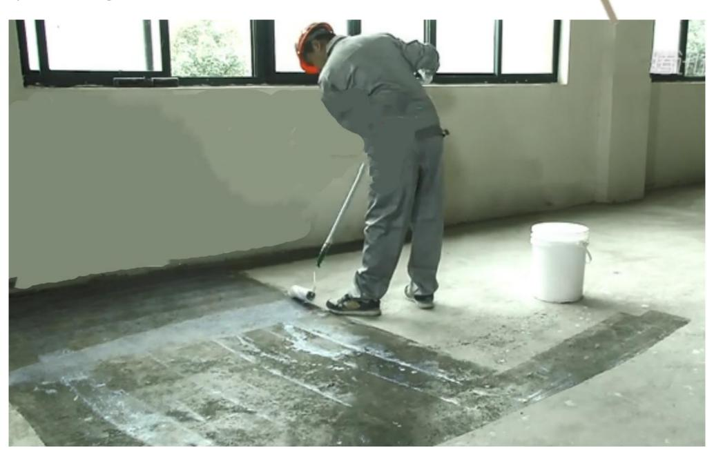
Constructing the interface primer should be uniform without obvious liquid accumulation. After it is dried, self-leveling construction can be carried out.
