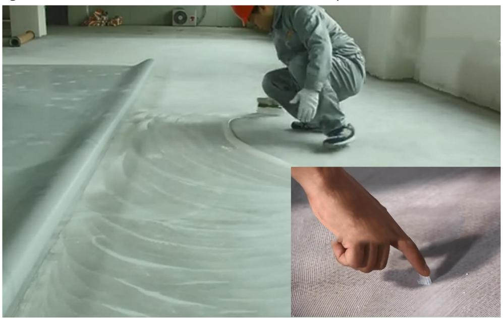
Rolling up one end of the flooring sheet, sweeping the ground and the back of the sheet, then using the appropriate scraping tooth coated adhesive on the ground, laying the floor later on.
